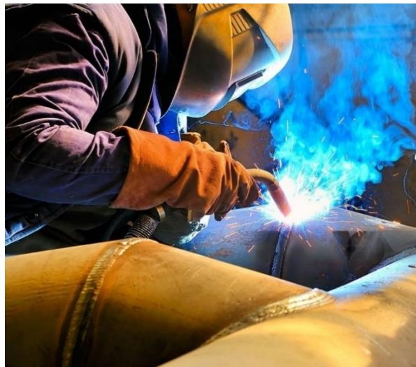
Figure 2 - Fumes and gases during welding.
